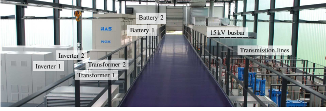
Fig. 2. Technology center of Younicos AG in Berlin with NaS Batteries, 500 kW inverters, transformers, transmission lines and 15 kV busbar.
