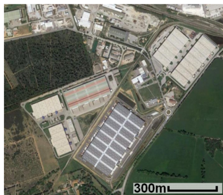
Figure 1. Optical image 28 of the warehouses used to illustrate the technique. The footprint of the picture is identical to the one in the radar images. North is up.
